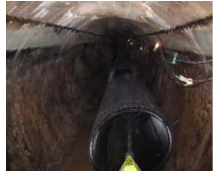
Figure 44. Etanchéité PEHD SURE GRIP
