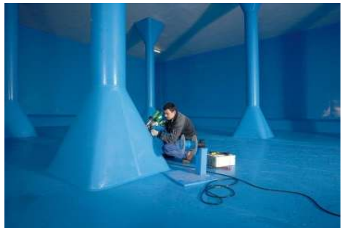
Figure 5. Habillage de poteaux
