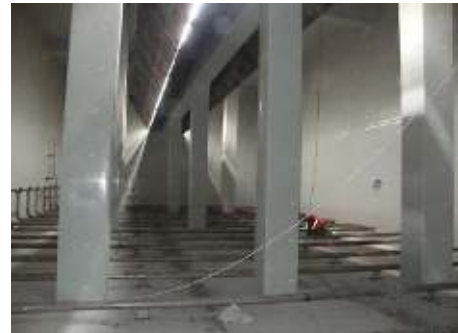
Figure 17. Habillage de poteaux
