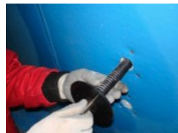
Figure 10. Ancrage PEHD
